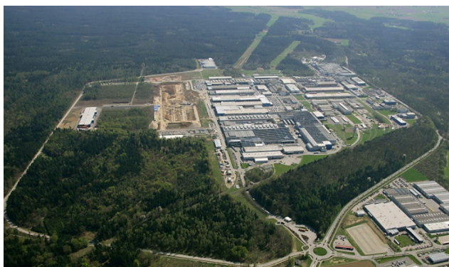
Picture 2: In the course of the AMAG 2014 large-scale project, AMAG's headquarters at Ranshofen are being expanded to become an even more technologically advanced, more profitable site. The overall project is one of the largest of its kind in the European aluminium industry.
