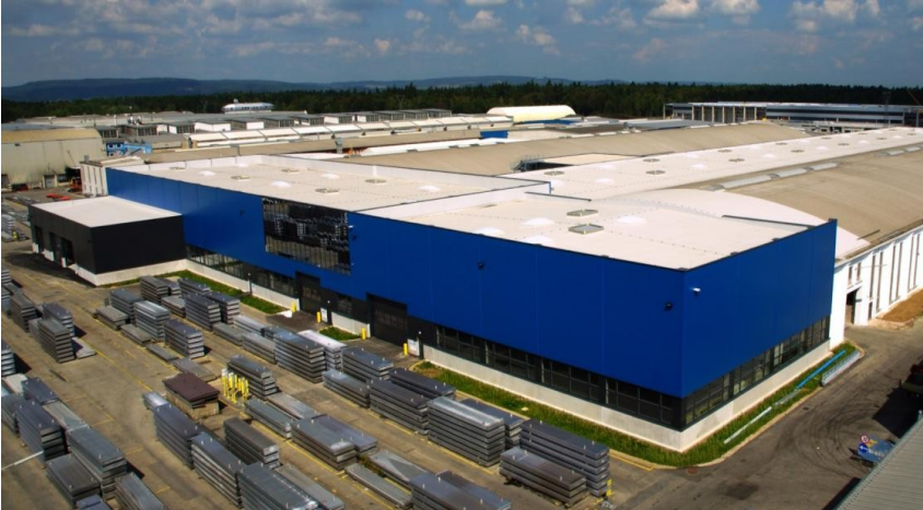
Construction work at new plate production centre completed
