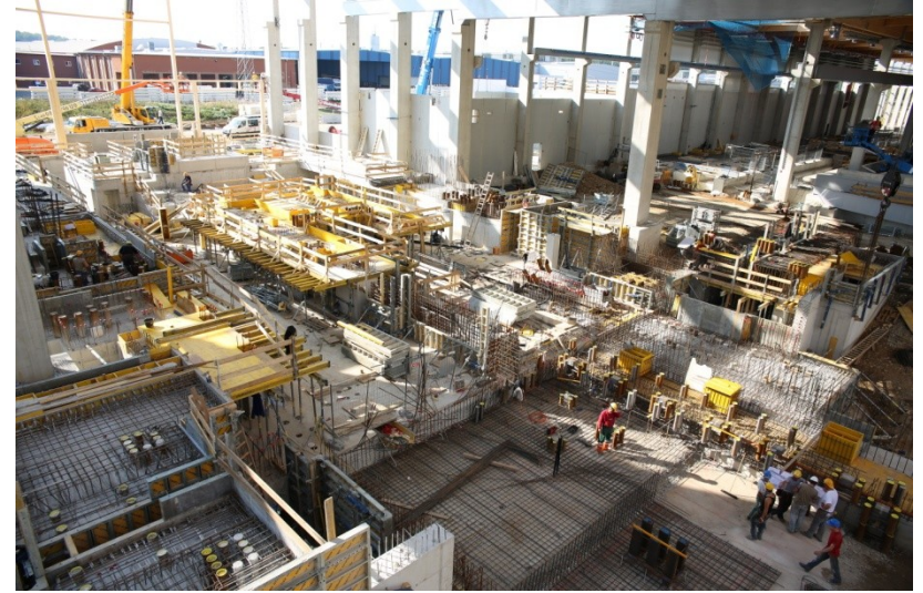
Foundation work at mill stand
