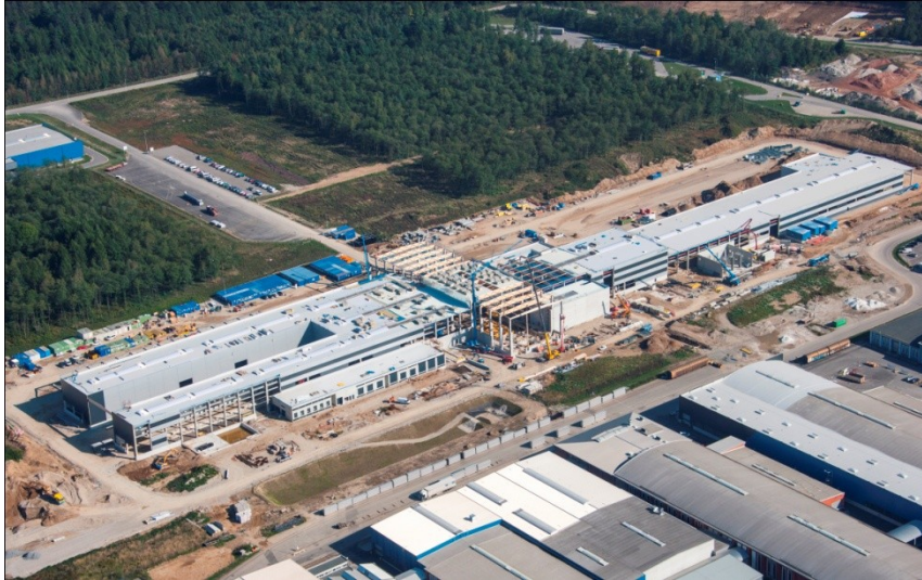
Significant progress on construction of rolling mill building
