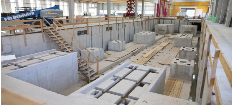
Foundation for the new plate stretcher as part of AMAG 2014
